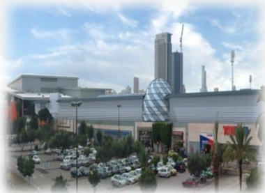
Azrieli Ayalon mall (additional floor) Approx. 9,500
