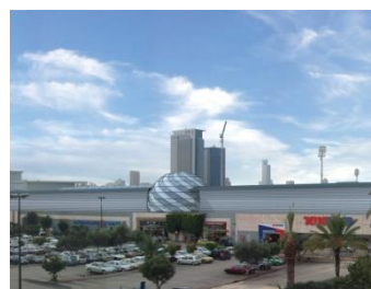
Azrieli Ayalon mall (additional floor) Approx. 9,500
