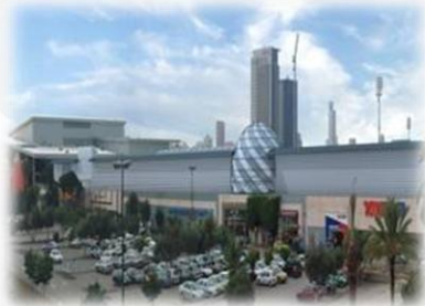
Azrieli Ayalon mall (additional floor) Approx. 9,500
