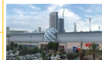
Azrieli Ayalon mall (additional floor) Approx. 9,500
