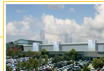
Azrieli Ayalon mall (additional floor) Approx. 9,500
