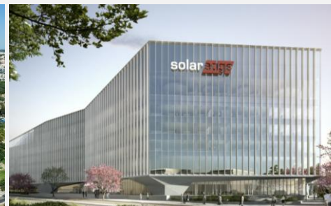
Ramat HaSharon SolarEdge ~43,000 m 2
